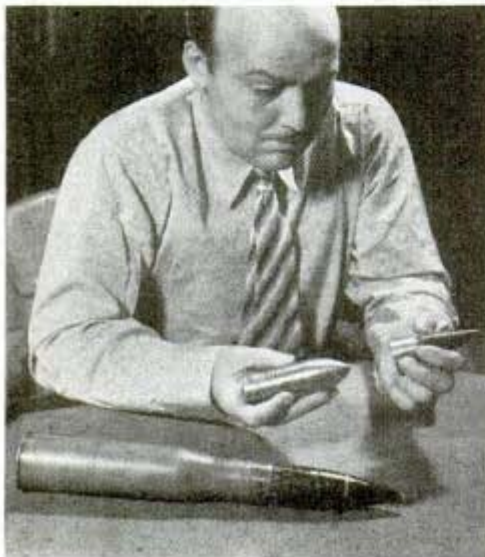
Dr. Bates shows how plastic nose fits onto projectile for an antitank weapon
